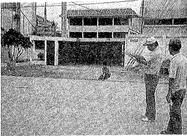
Checking of Road Width
