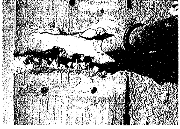
Photo - 5 Water Seal of Center Support Column (Goaze STP)
