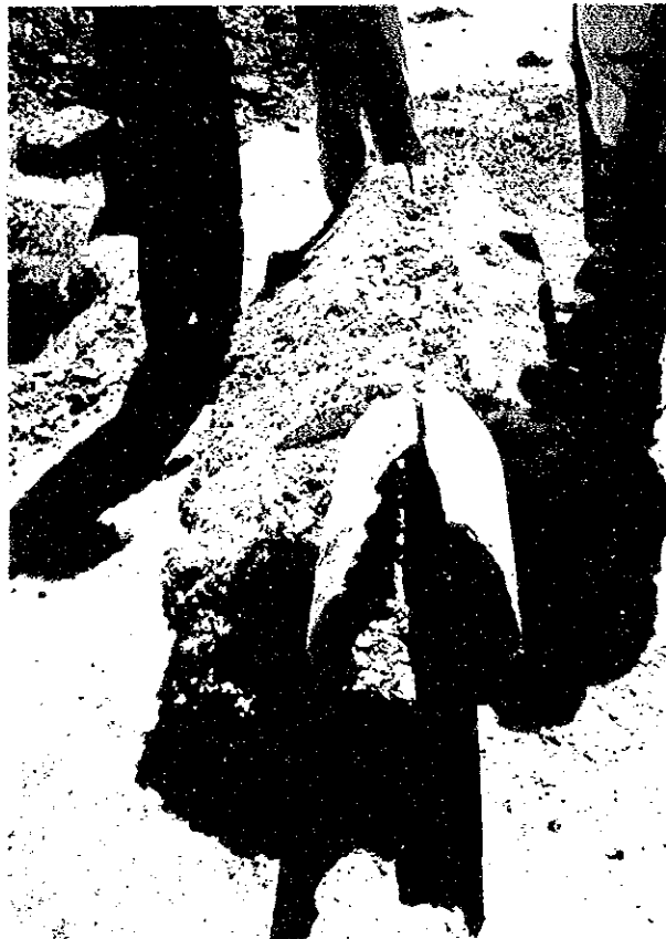
Photo - 2 Broken Rising Main
