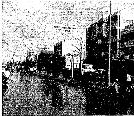
Urban Section of Six-lane National Highway (Rt. 3 Changwat Rayong)
