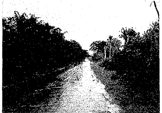
DBST pavement in "fair" condition N5-1: Tagbilaran-Cortes
