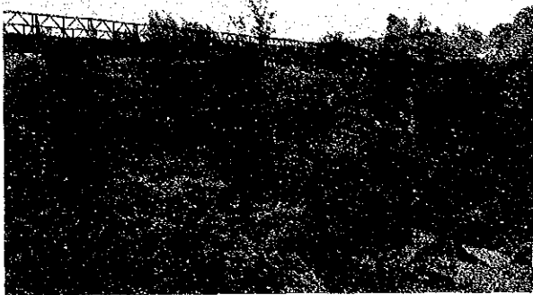
Bailey bridge over the deep valley P27-1: Magallanes-Maragondon, Provincial road, Cavite
