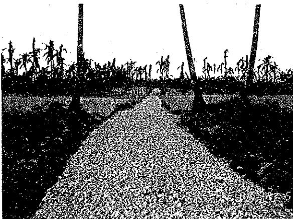
Newly constructed gravel road B8-3: Gaid-Divisoria
