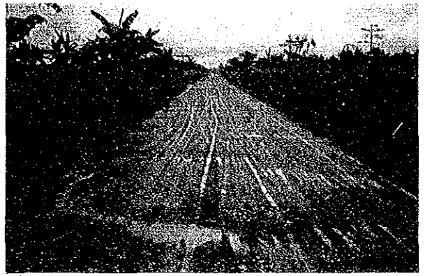
Gravel road in "bad" condition N11-1: Jct. Tiniwisan-Maguinda
