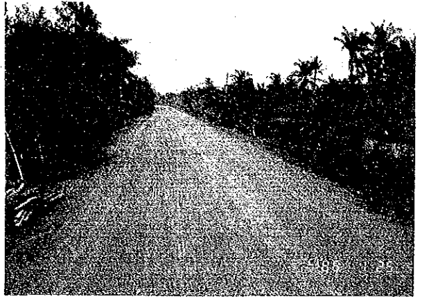
Gravel road in "fair" condition N9-3: Malinta-Milagros
