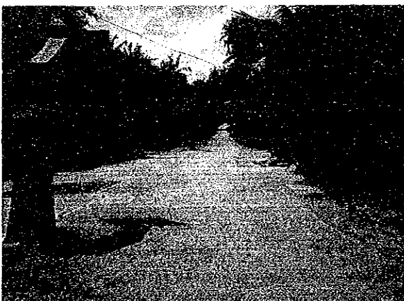
PCC pavement at the barangay center is used for multipurpose B28-5: Taug Barangay Road
