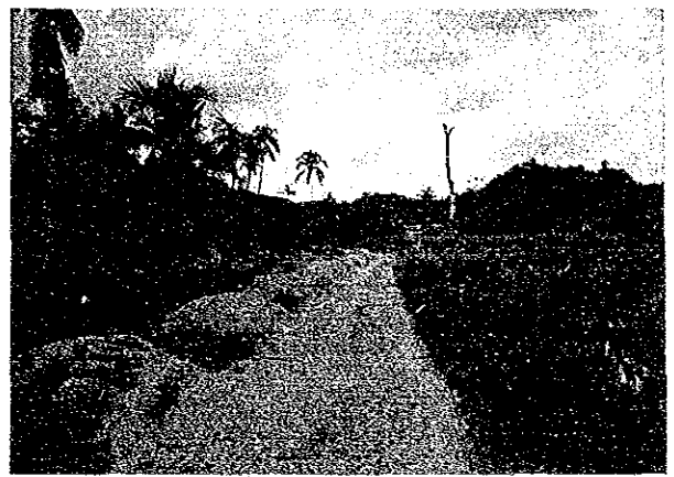
Gravel road in "very bad" condition P80-1: Canmanico-Anonang
