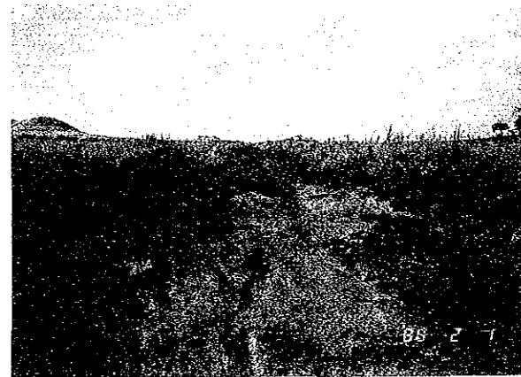
Earth road in "very bad" condition P25-1: Jct. Bangad-Bangad
