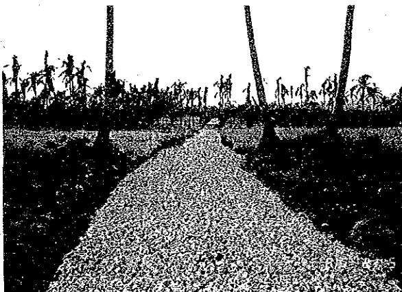
Newly constructed gravel road B8-3: Gaid-Divisoria
