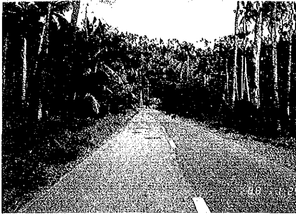
DBST pavement in "fair" condition N9-1: Masbate-Malinta
