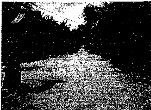
PCC pavement at the barangay center is used for multipurpose B28-5: Taug Barangay Road
