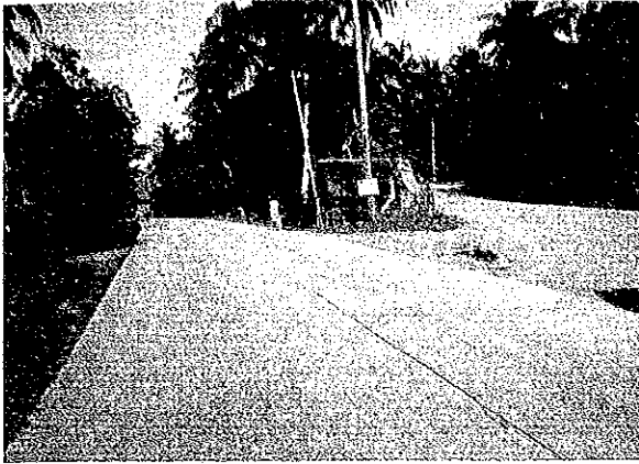
PCC pavement in "good" condition N5-3: Cortes-Jct. Antequera
