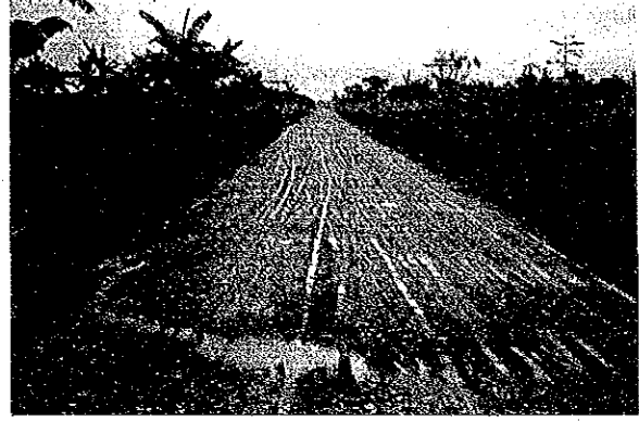
Gravel road in "bad" condition N11-1: Jct. Tiniwisan-Maguinda
