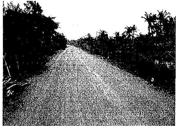
Gravel road in "fair" condition N9-3: Malinta-Milagros
