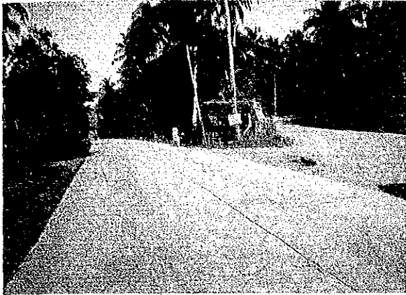
FCC pavement in "good" condition N5-3: Cortes-Jct. Antequera
