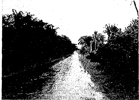
DBST pavement in "fair" condition N5-1: Tagbilaran-Cortes
