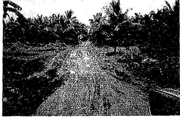
Gravel road in "very bad" condition P4-76: Jobanga-Badiang
