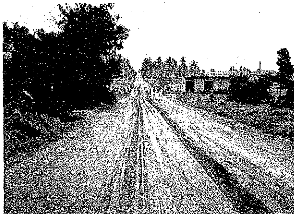
Gravel road in "fair" condition P108-1: Guindulman-Anda
