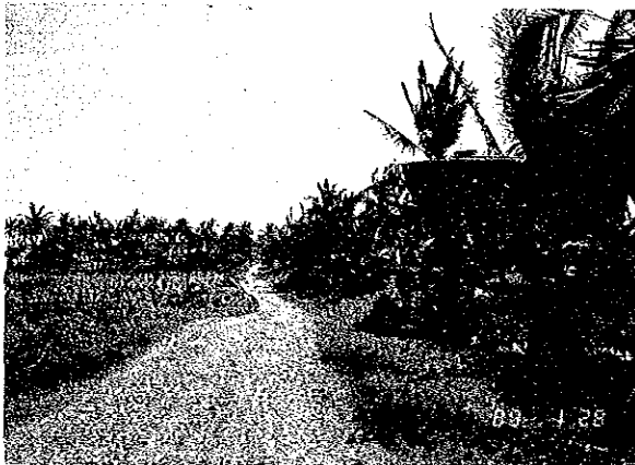
Gravel road in "bad" condition P31-1: Curvada-Pio V. Corpus
