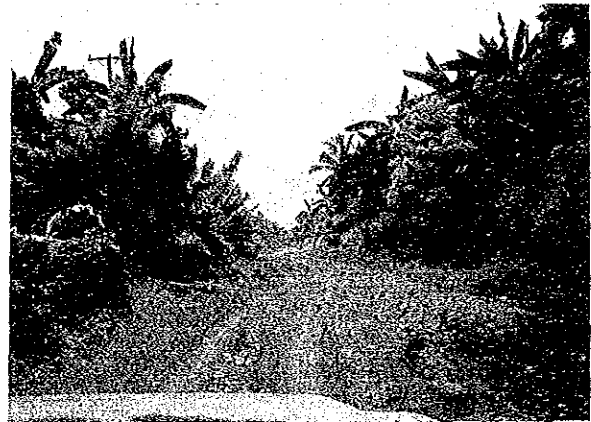
Gravel road in "very bad" condition P29-1: Alfonso-Maragoñdon
