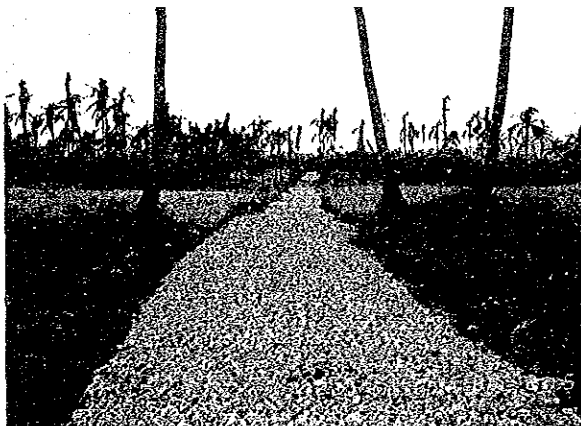
Newly constructed gravel road B8-3: Gaid-Divisorja
