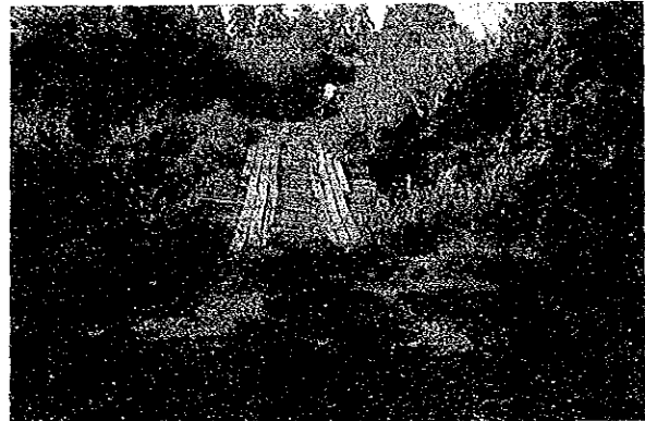
Dilapidated timber bridge P6-43: Jct. T-Maguinda-Lasnieves, Provincial road, Agusan del Norte
