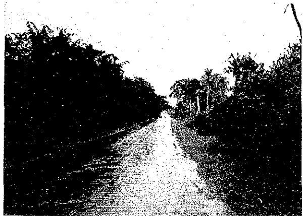
DBST pavement in "fair" condition N5-1: Tagbilaran-Cortes
