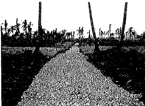
Newly constructed gravel road B8-3: Gaid-Divisorja
