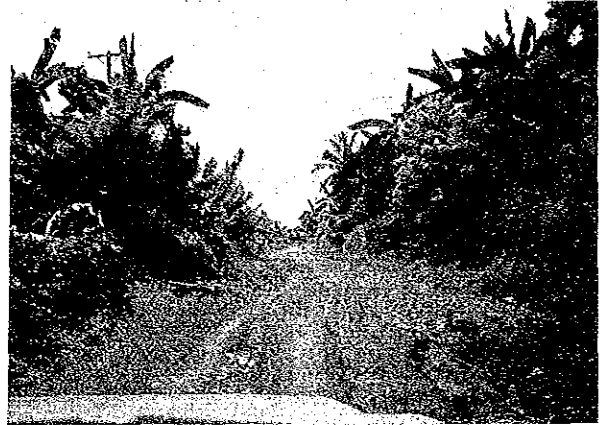
Gravel road in "very bad" condition P29-1: Alfonso-Maragondon
