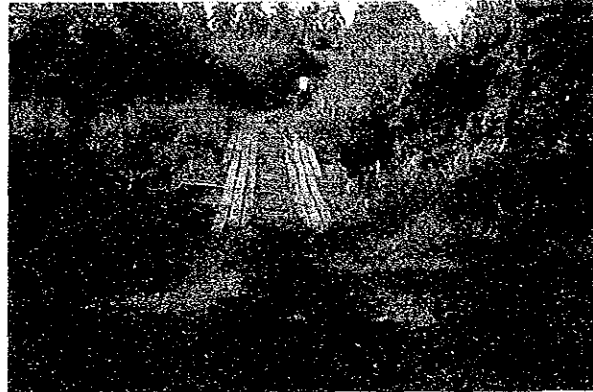
Dilapidated timber bridge P6-43: Jct. T-Maguinda-Lasnieves, Provincial road, Agusan del Norte
