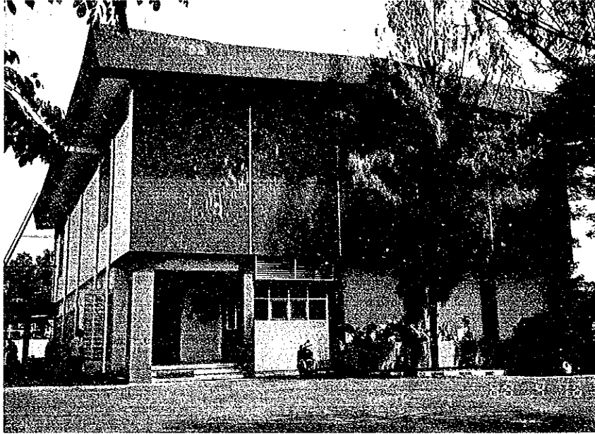
CAW Switching Center
