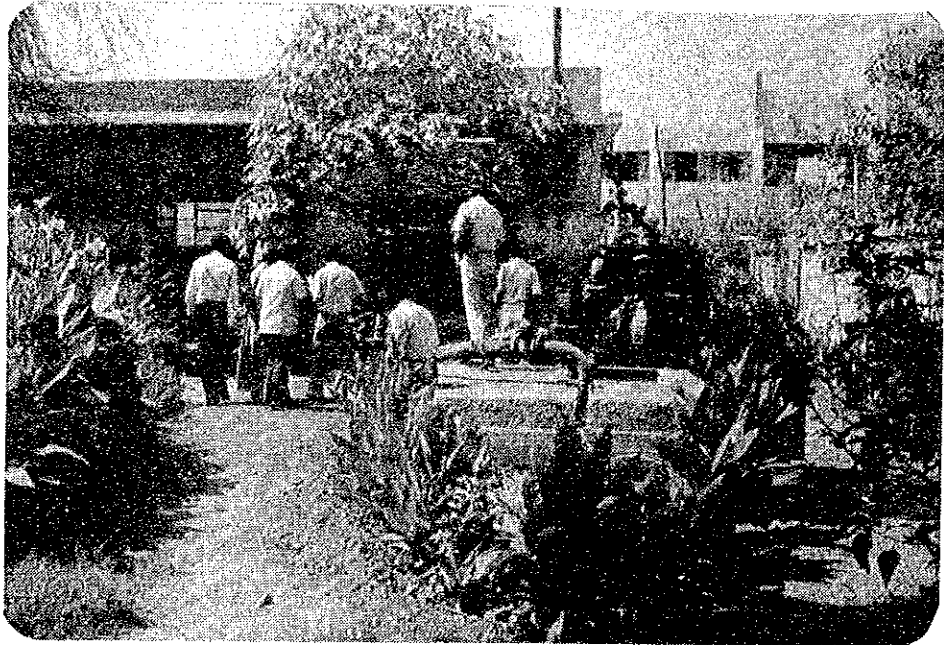
Photo 2.6 Sanawiya Pumping Station (Bilbeis)
