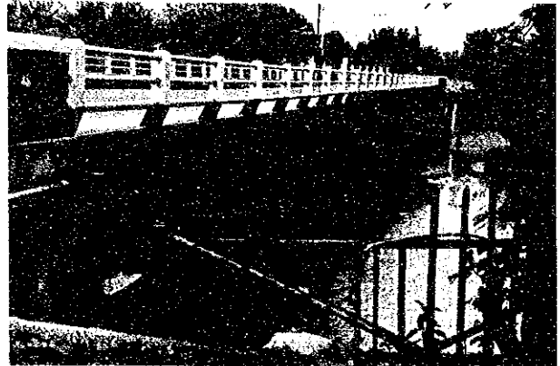
Gilampeni Bridge near Marugahayu
