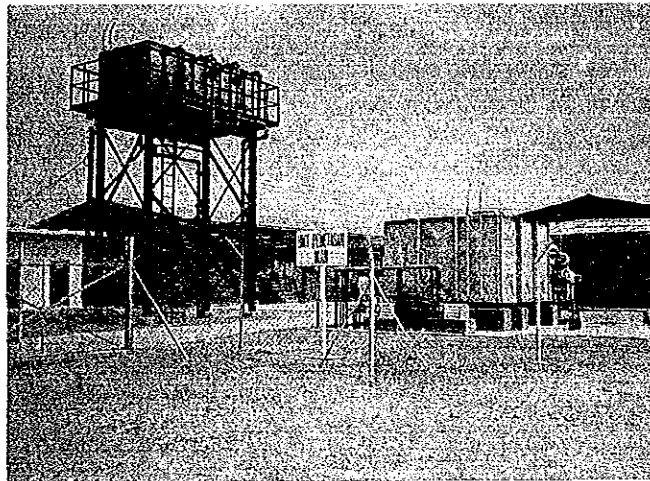
Figure 8. Water Filtration System showing the water treatment tanks and the water storage tank.
