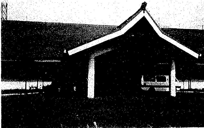
No.2 Main Building of CDAET
