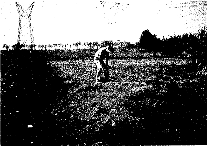
No.10 Bearing Capacity Survey with Cone Penetrometer
