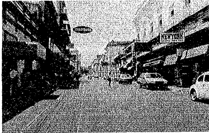
PHOTO 3-6-3 COMMERCIAL SIGN BOARDS OVER THE STREETS
