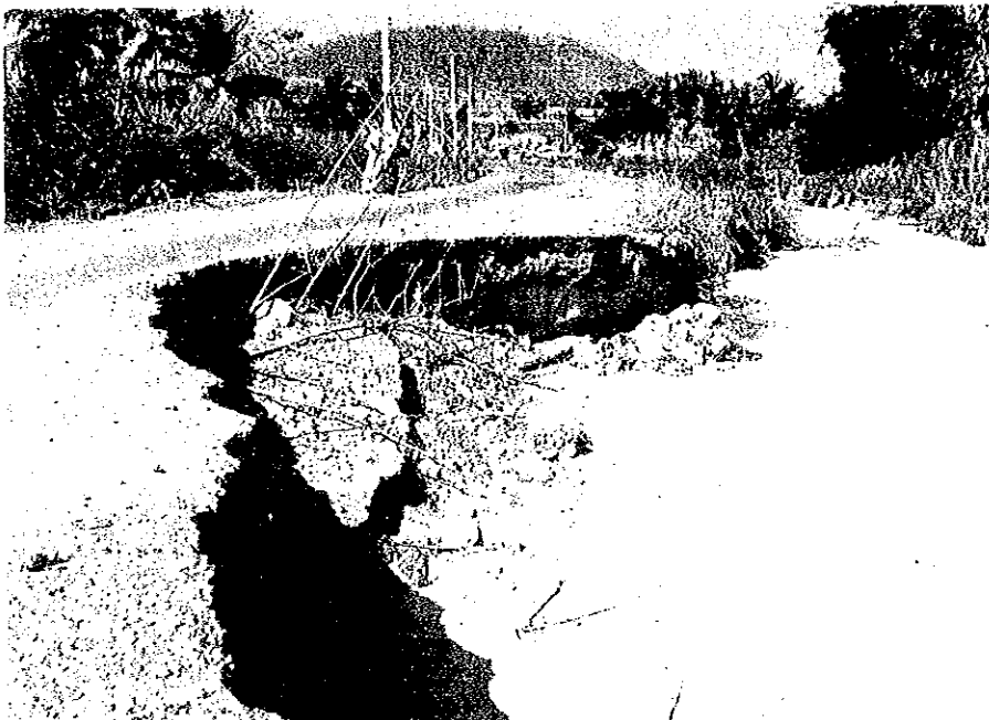
Road collapse caused by erosion
