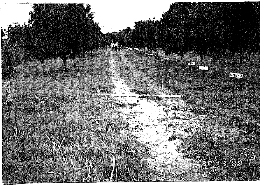
No.5 Existing Secondary Farm Road
