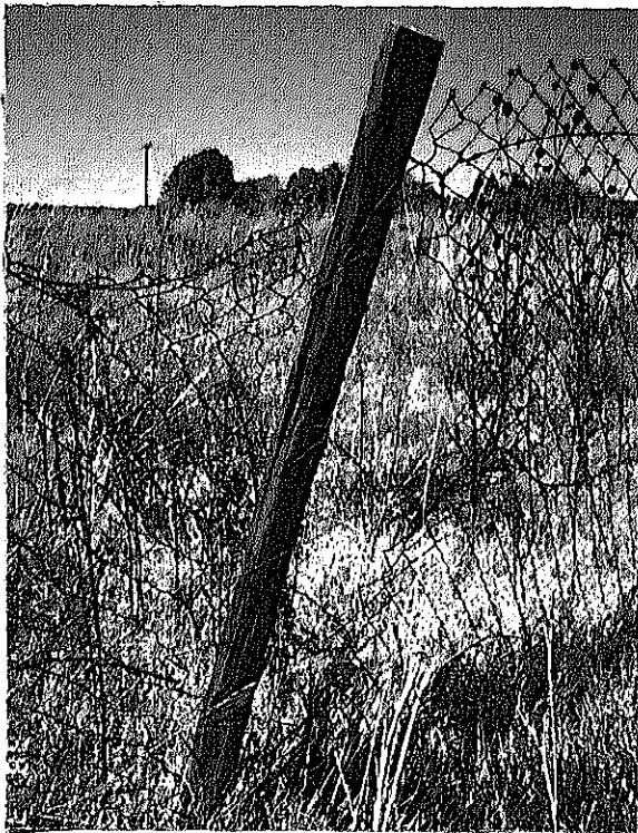
No.8 Existing Fence
