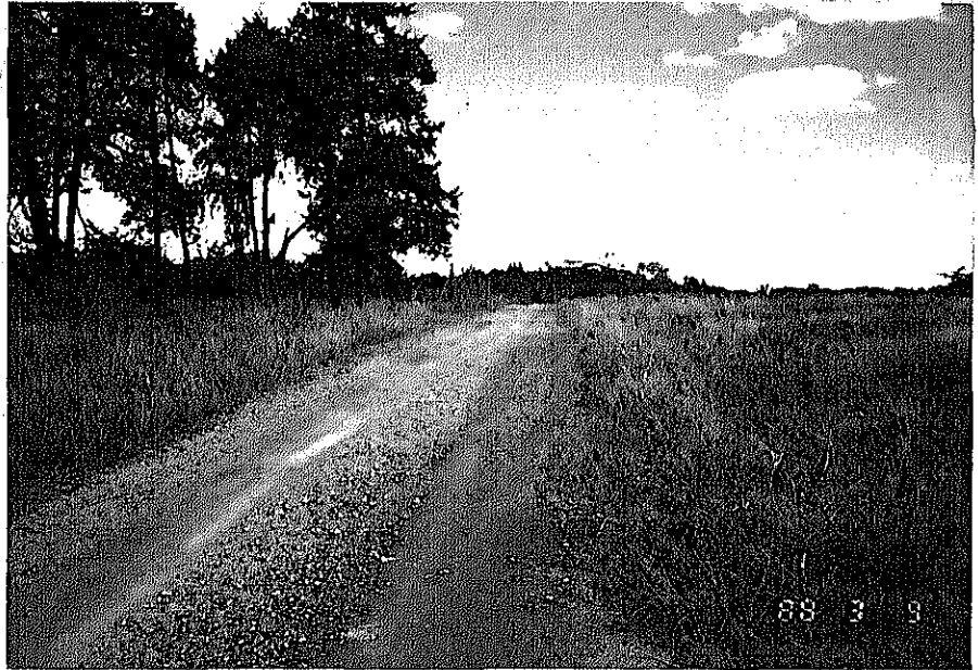
No.4 Existing Main Farm Road
