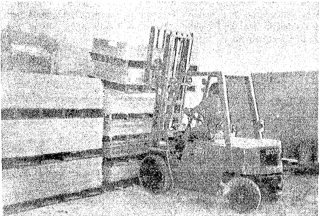
Storage of the completed pulp cement boards
