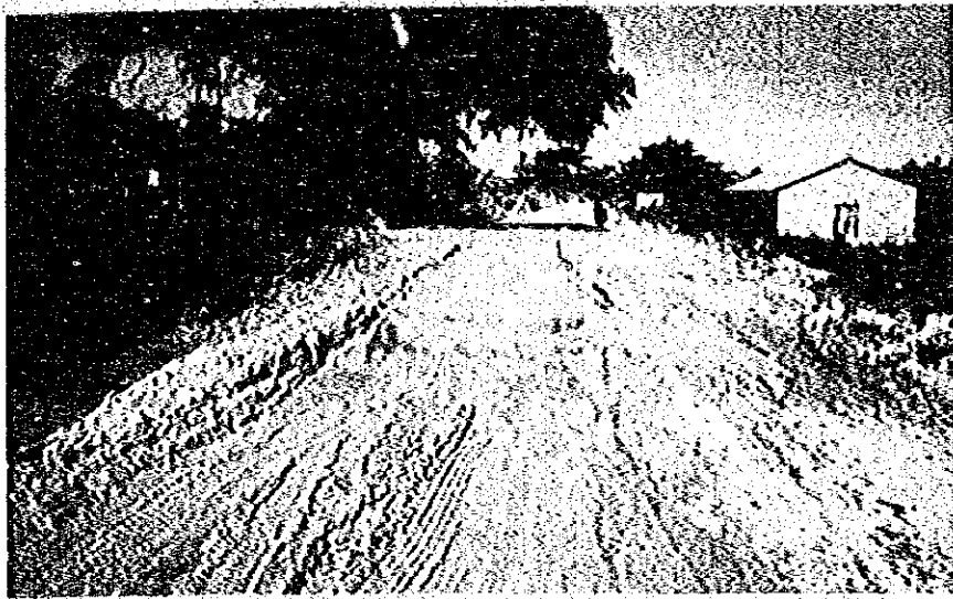
Road to be improved with cross drain(Iringa Kilolo)
