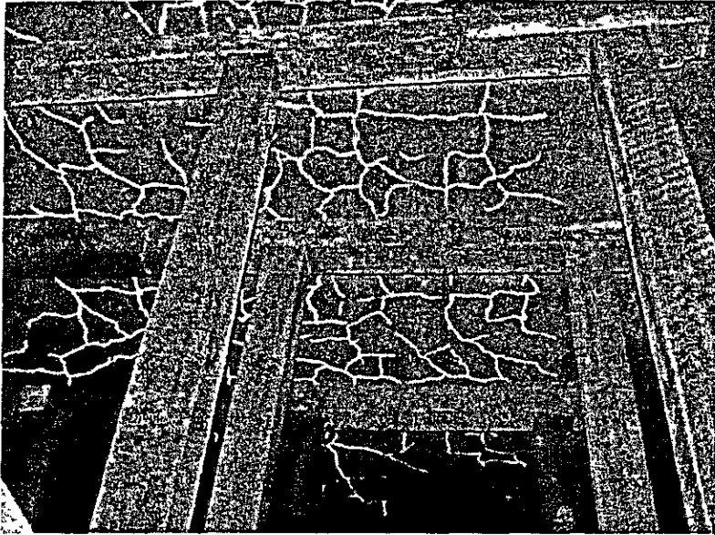
Photo 3-8.5 Cracks and Timberings under the RC Slab at the 6 Spans Continuous RC Rigid Bridge (B.K.K Side)
