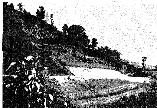
Concrete frame crib wall constructed as the countermeasure for large landslide of cut slope.
