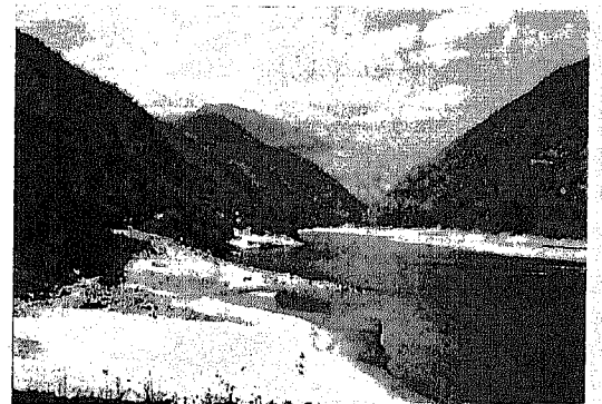
The route runs on the right bank of Sun Kosi river in the section between Khurkot and Nepithok.
