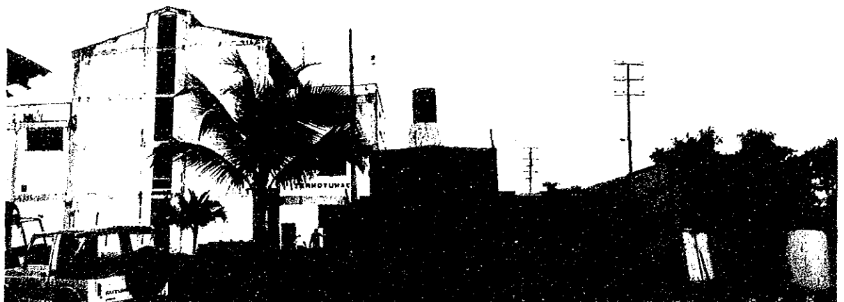
TERMOTUMACO POWER PLANT IN NARIÑO Department (No. 1 and 2 unit are installed in Building. No. 3 and 4 unit are outdoor packages.)
