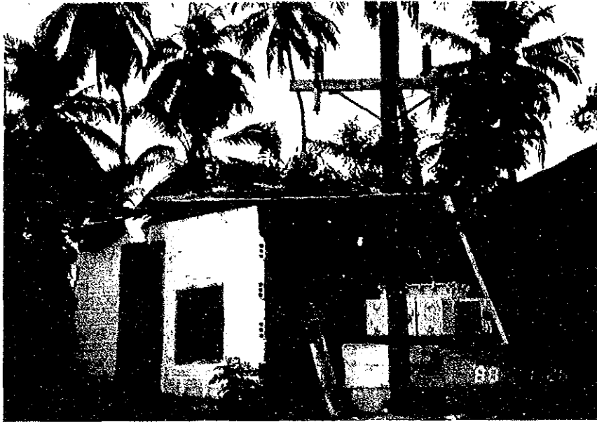
CAPURGANA POWER PLANT IN CHOCO Department
