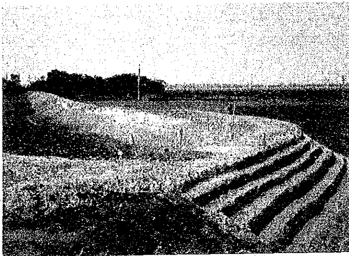
Main Irrigation Canal Embankment nearby Barba Village (under reinforcement work by BWDB)
