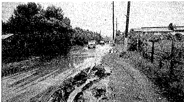
Road whose surface elevation is around zero meter. (Malabon area)
