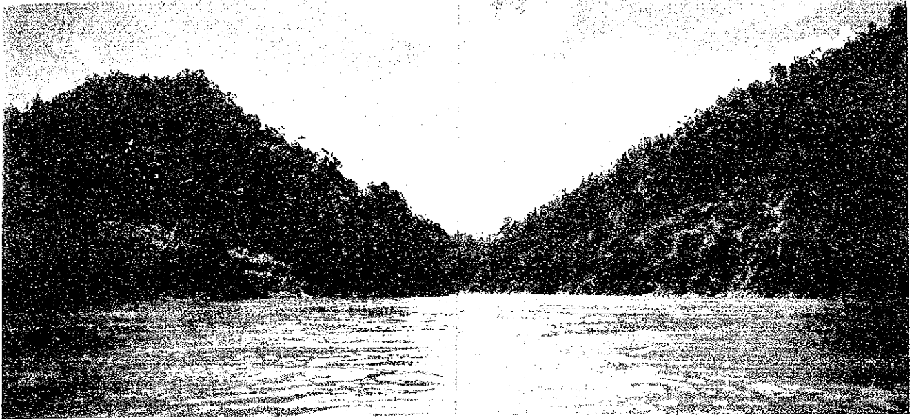
Dabong Dam site
