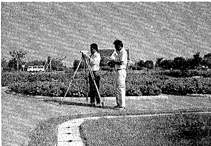
Checking of height (AUTO LEVEL AE)
