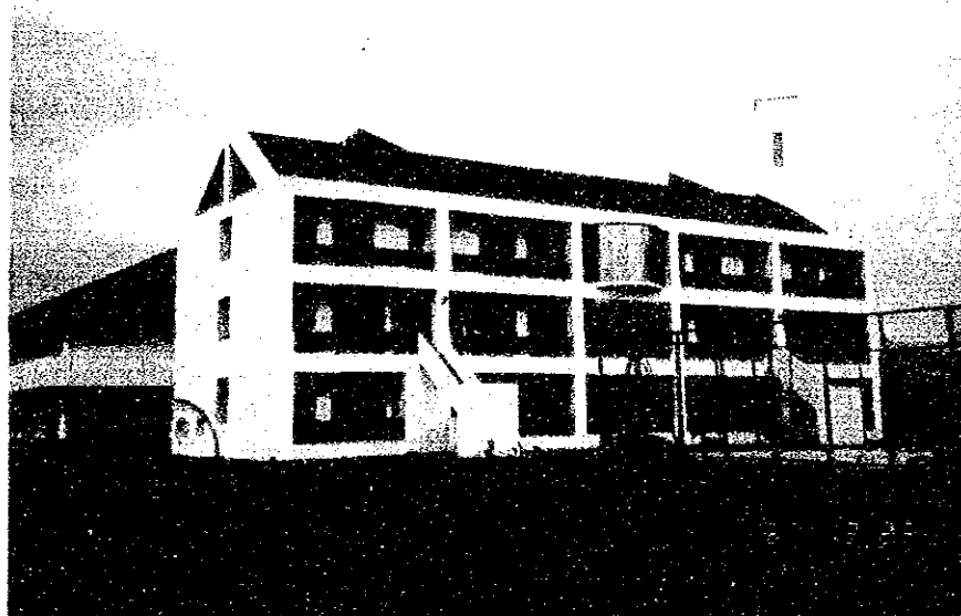
No.4 Dormitory of Jatisari Center ( Reinforced Concrete, three-storied Building )
