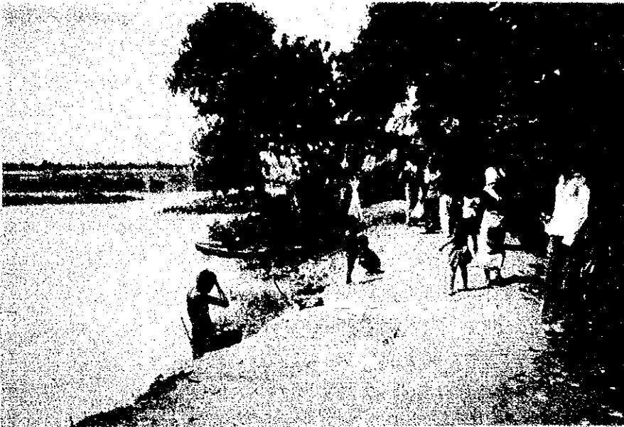
(J) Existing road along Lakhya River in southern part of the Project area (near Ghandarbapur)
