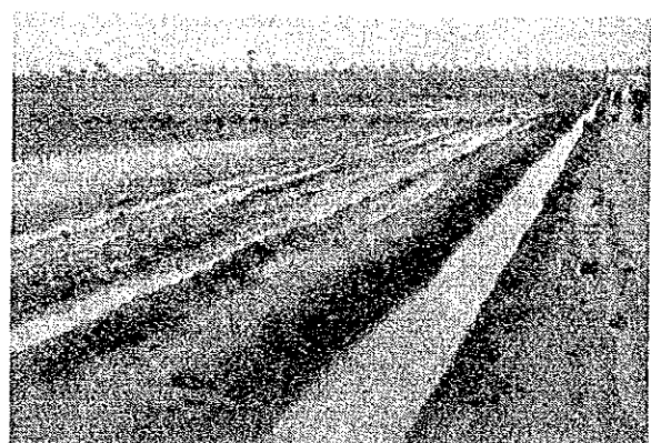
Completed paddy fields and canal
