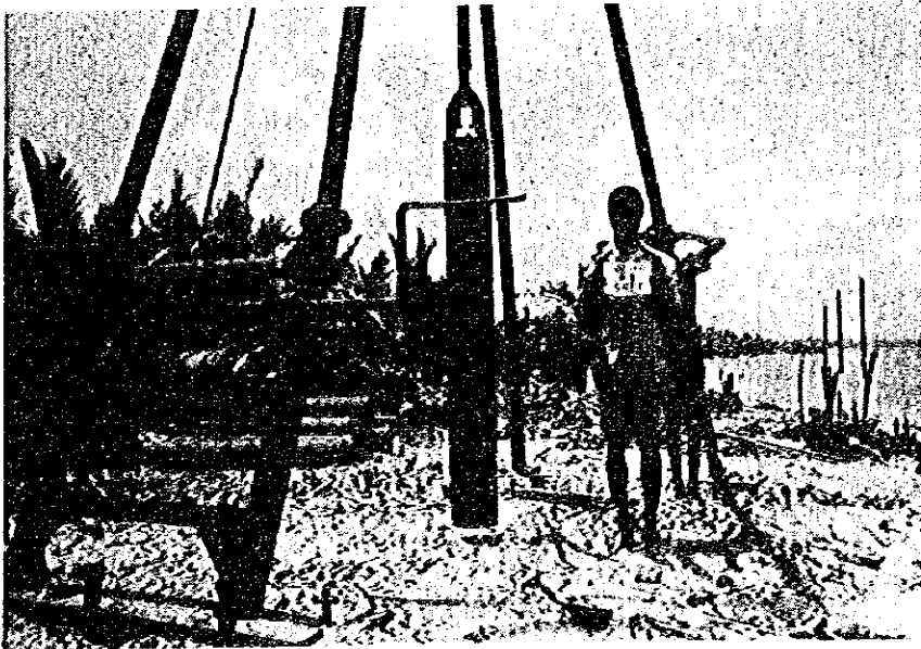
Start to Drill by Manual Type Boring Machine at 0-2
