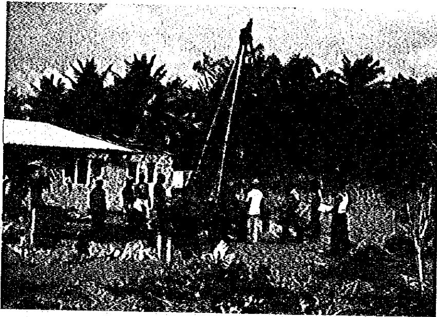
Motor-driven boring machine (1/4)
