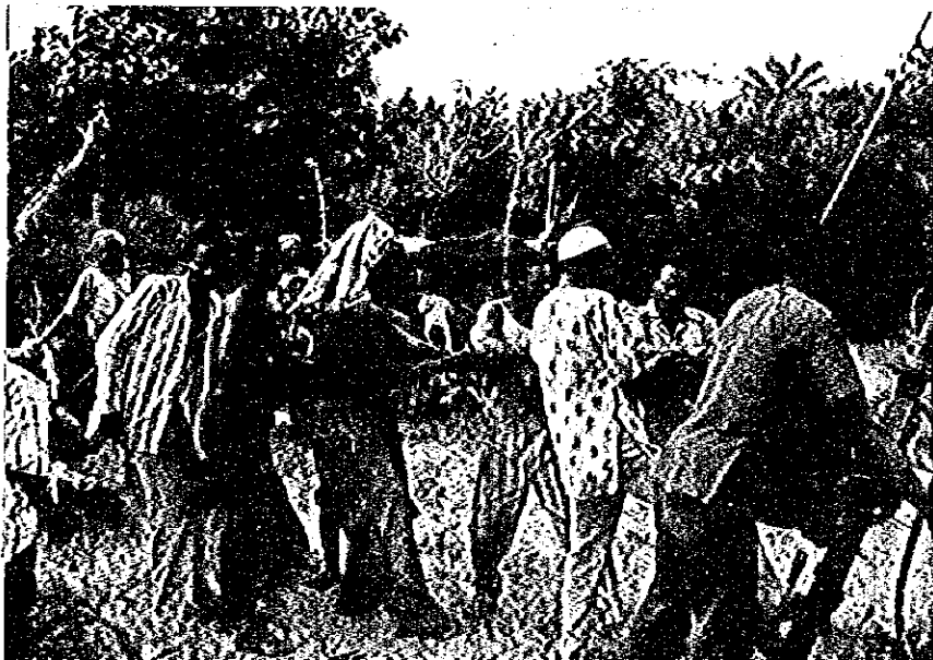
Operation of manual-type boring machine
