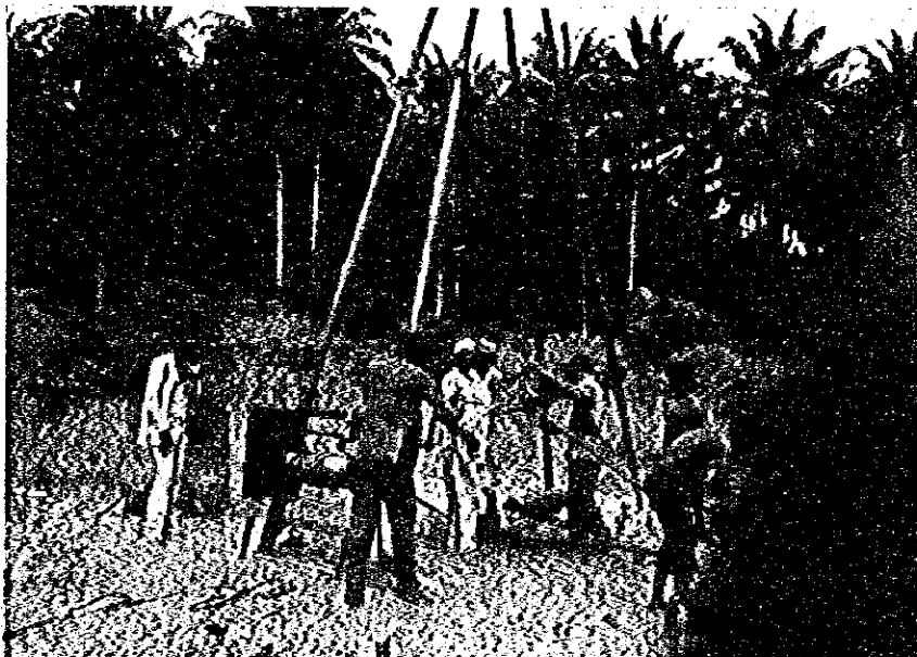
Manual-type boring machine (1/2)
