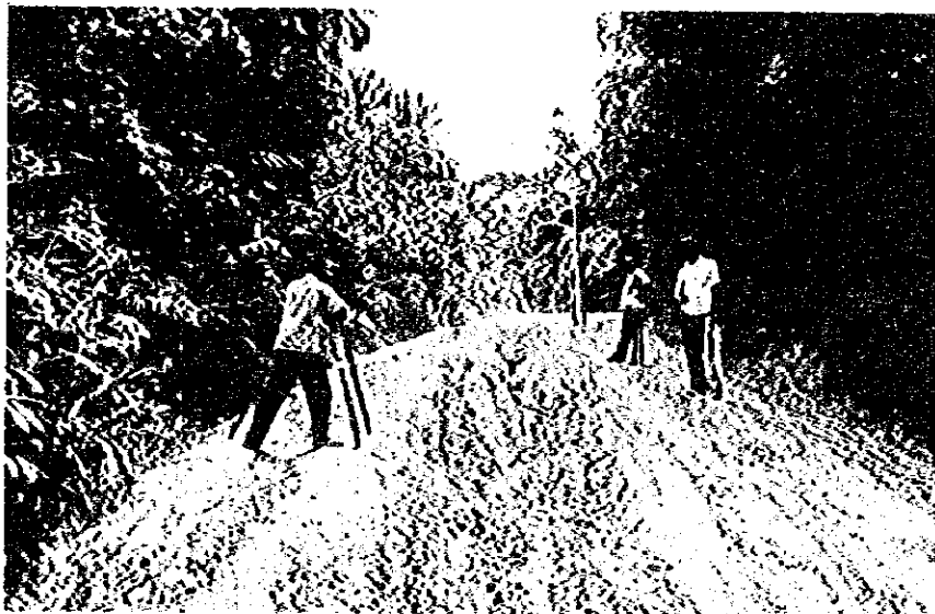
LISCO ROAD IN POOR CONDITION
