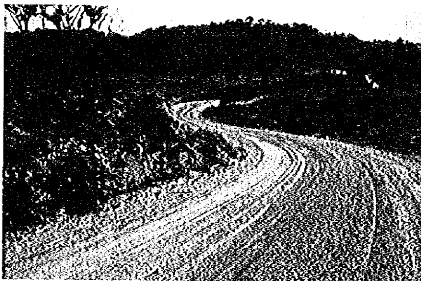
LATERITE-PAVED ROAD IN GBARNGA-VOINJAMA SECTION
