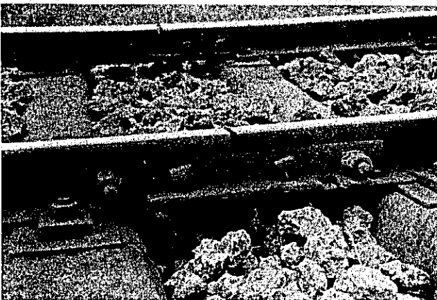
Picture 4-3. Ballast and joints of rails
