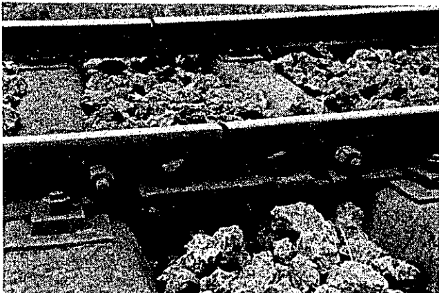
Picture 4-3. Ballast and joints of rails
