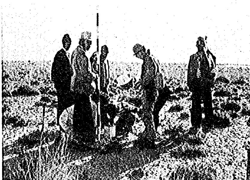
Photo. 3 Gravity Survey and Leveling Survey in the Field
