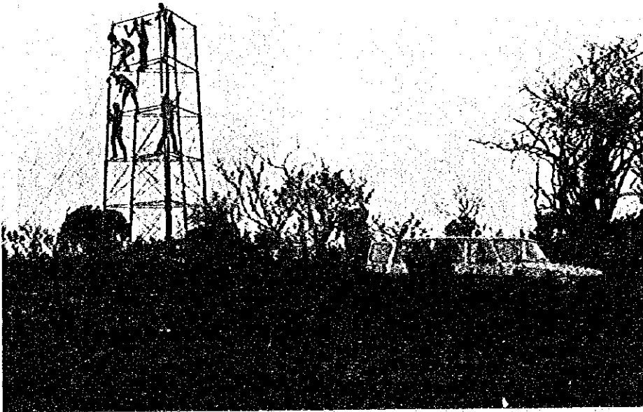
Construction of observing tower.
