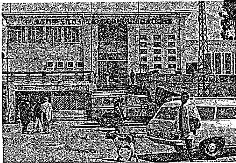
Fig 90 View of DESSIE Telephone Office
