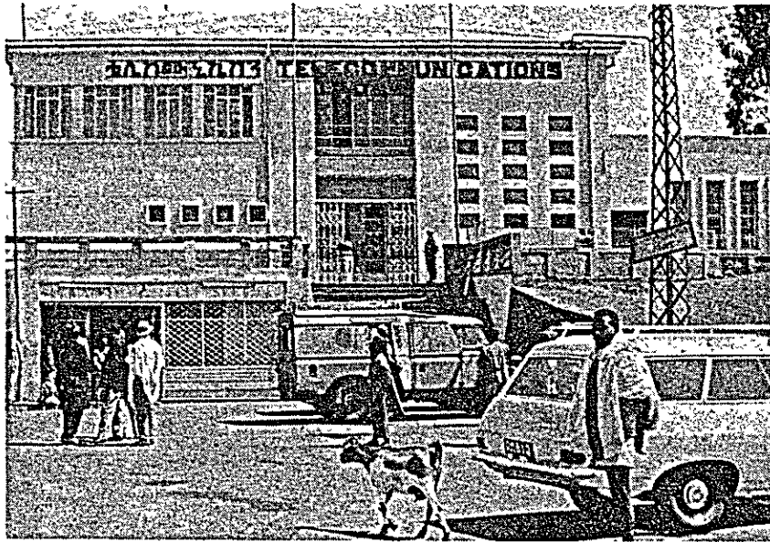
Fig. IV-33 View of Telephone Office of Dessie City
