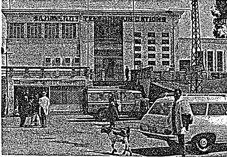
Fig. 90 View of DESSIE Telephone Office
