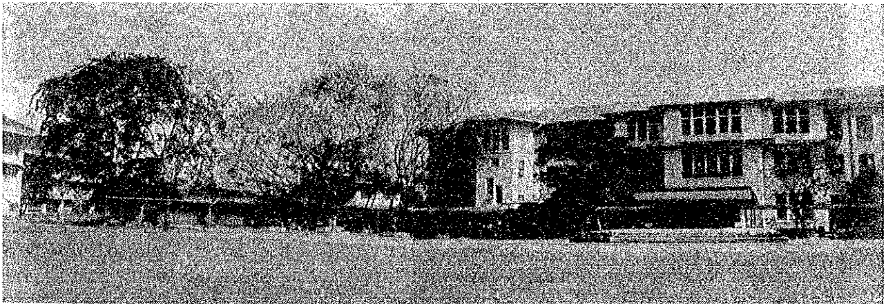
Campus (on the side of the project area)
