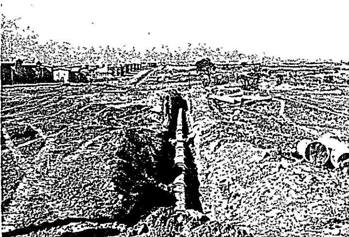
View of distribution pipe line, under con- struction in Islamabad
