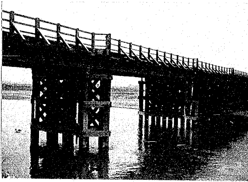
Road Bridge between Biratnagar and Itahari
