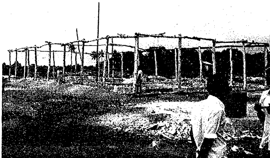
Picture No. 2 Temporary Work
