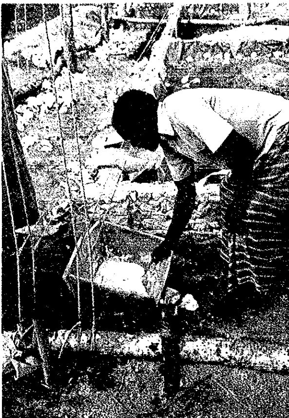
Picture No. 3 Stone Masonry and Mason
