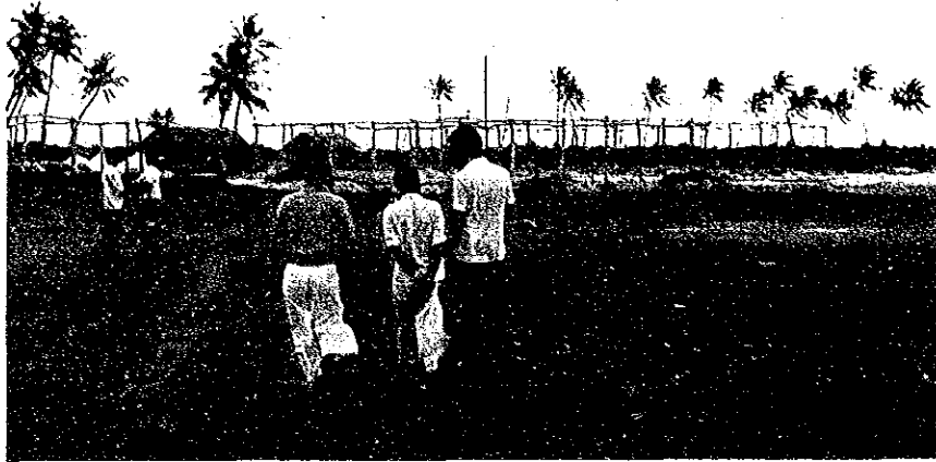
Picture No. 1 Temporary Housing and Scaffolding
