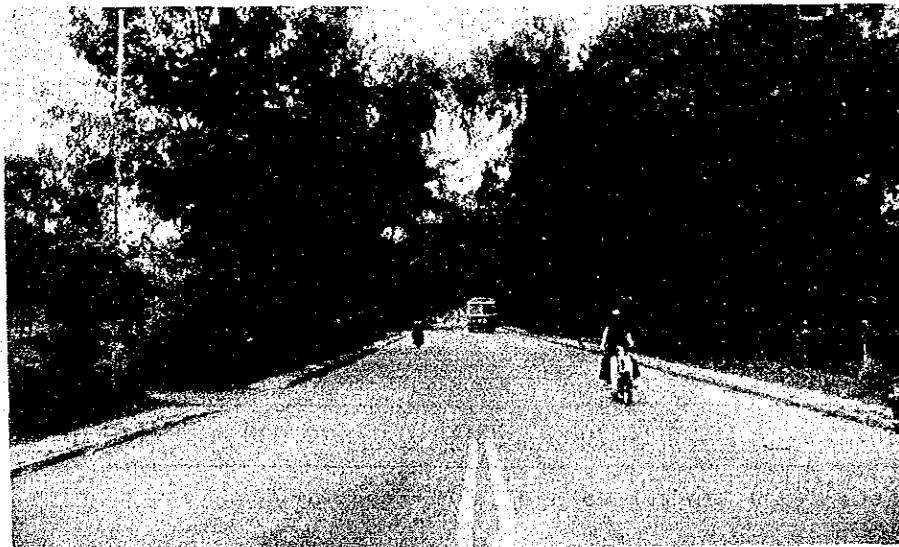
Typical Wide Single Carriage-Way
