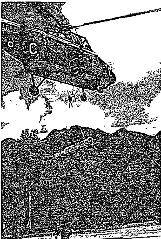
PHOTO 3. ANTENNA MAST CARRIED TO GUNONG SERAPI STATION BY A HELICOPTER
