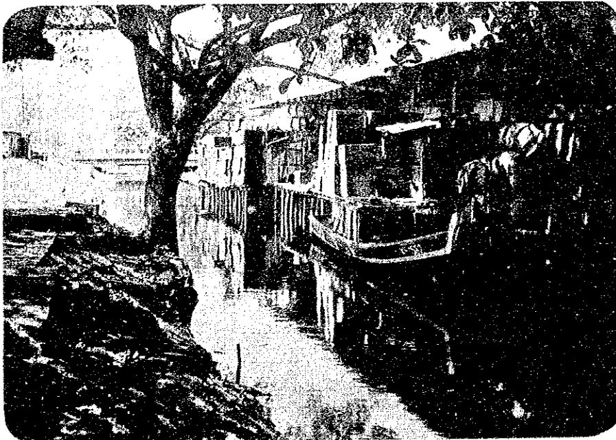
Photo 2 Trunk drain at Jl. Sungai Korok
