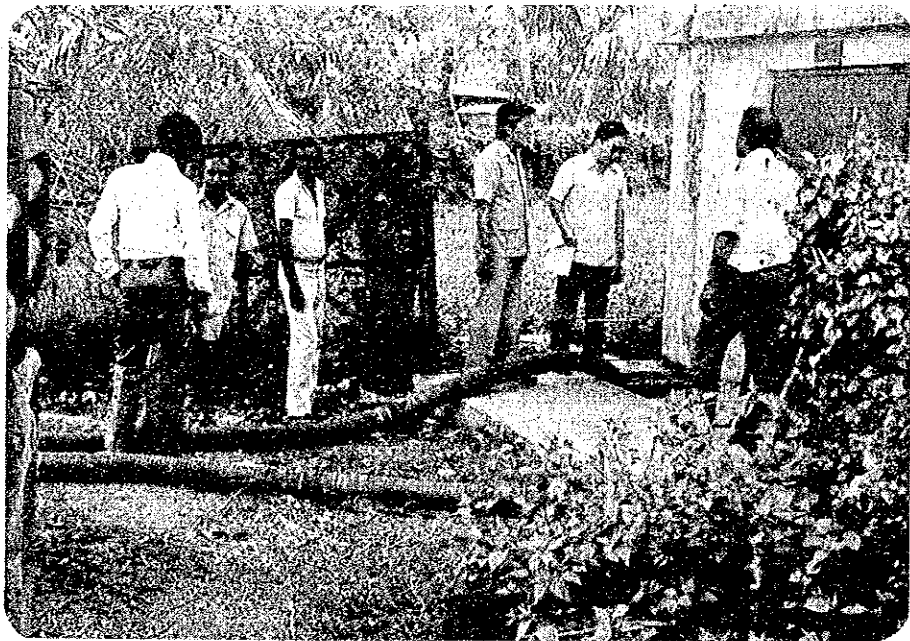
Photo 6 Suction hose of tank lorry
