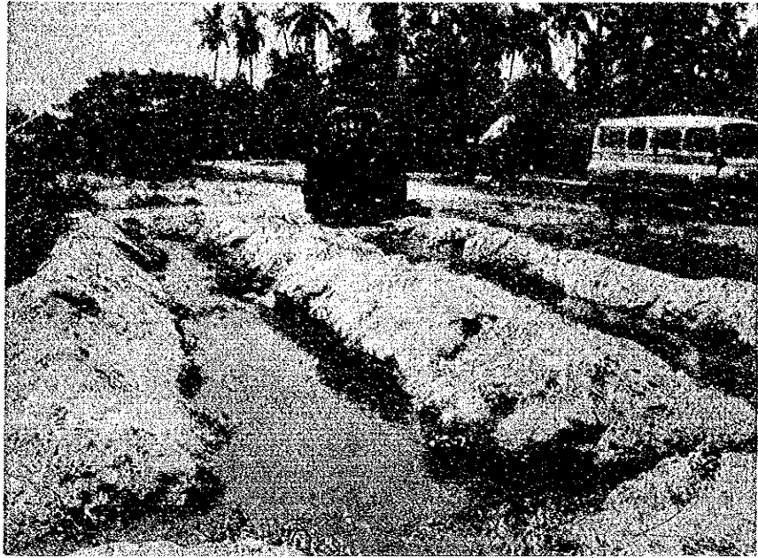
V-trenches for sludge dumping
