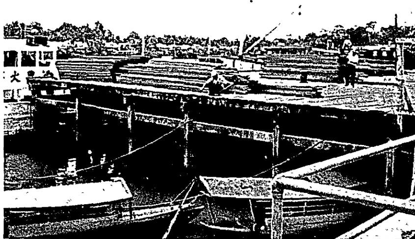
PIER FOR COASTAL VESSELS
