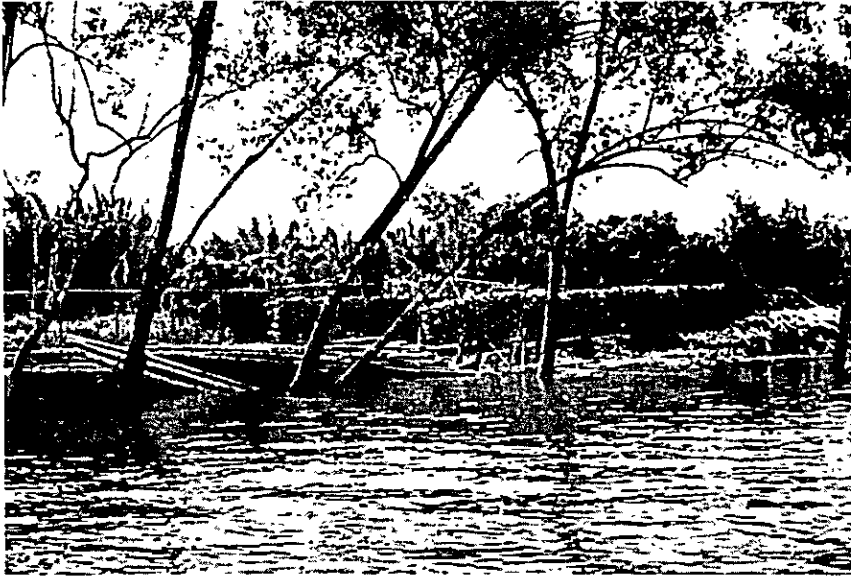
DOWN STREAM OF PENDING CUSTOMS : EROSION
