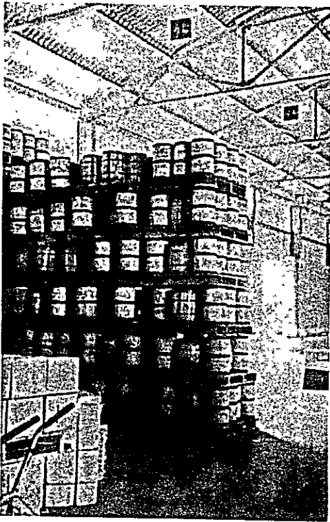
INSIDE OF THE TRANSIT SHED
