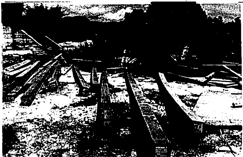
Photo.7-3 Curved Timber Piles
