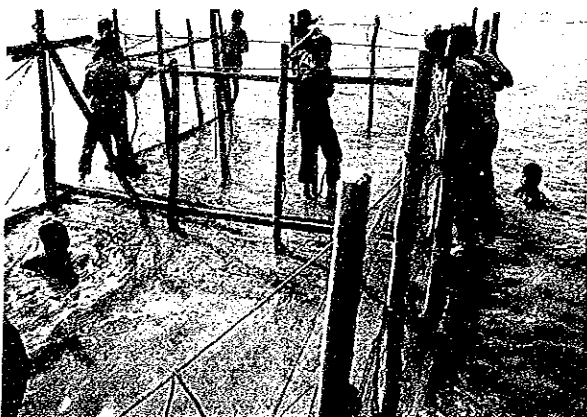
Photo 37 Construction of fish pen
