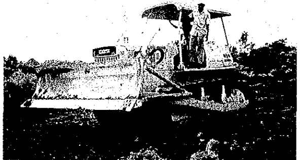
Site preparation for yellow fire belt
